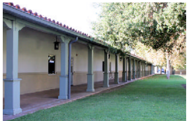
Several classroom buildings remain along with the outdoor corridors.
